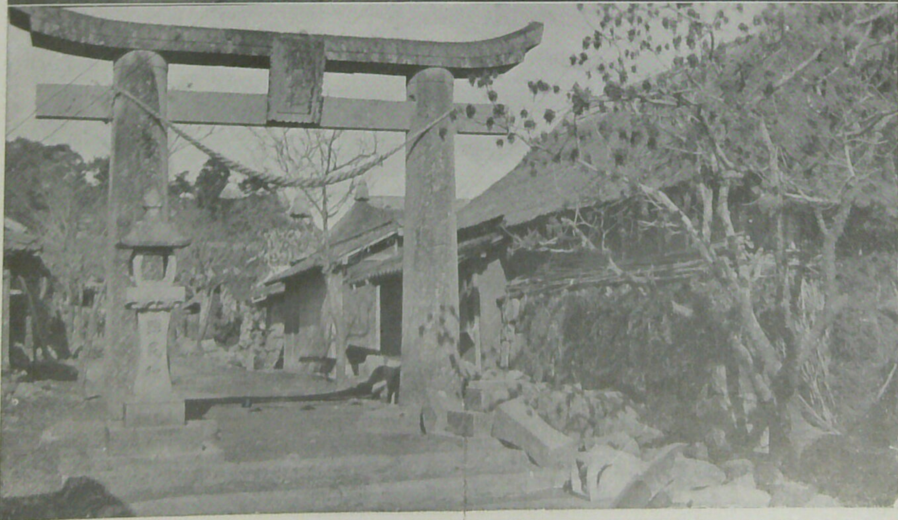
A Torii at Higashi-Arie displaced as much as 5 cm. One of a pair of stone lanterns in front overturned and the other remained intact.
