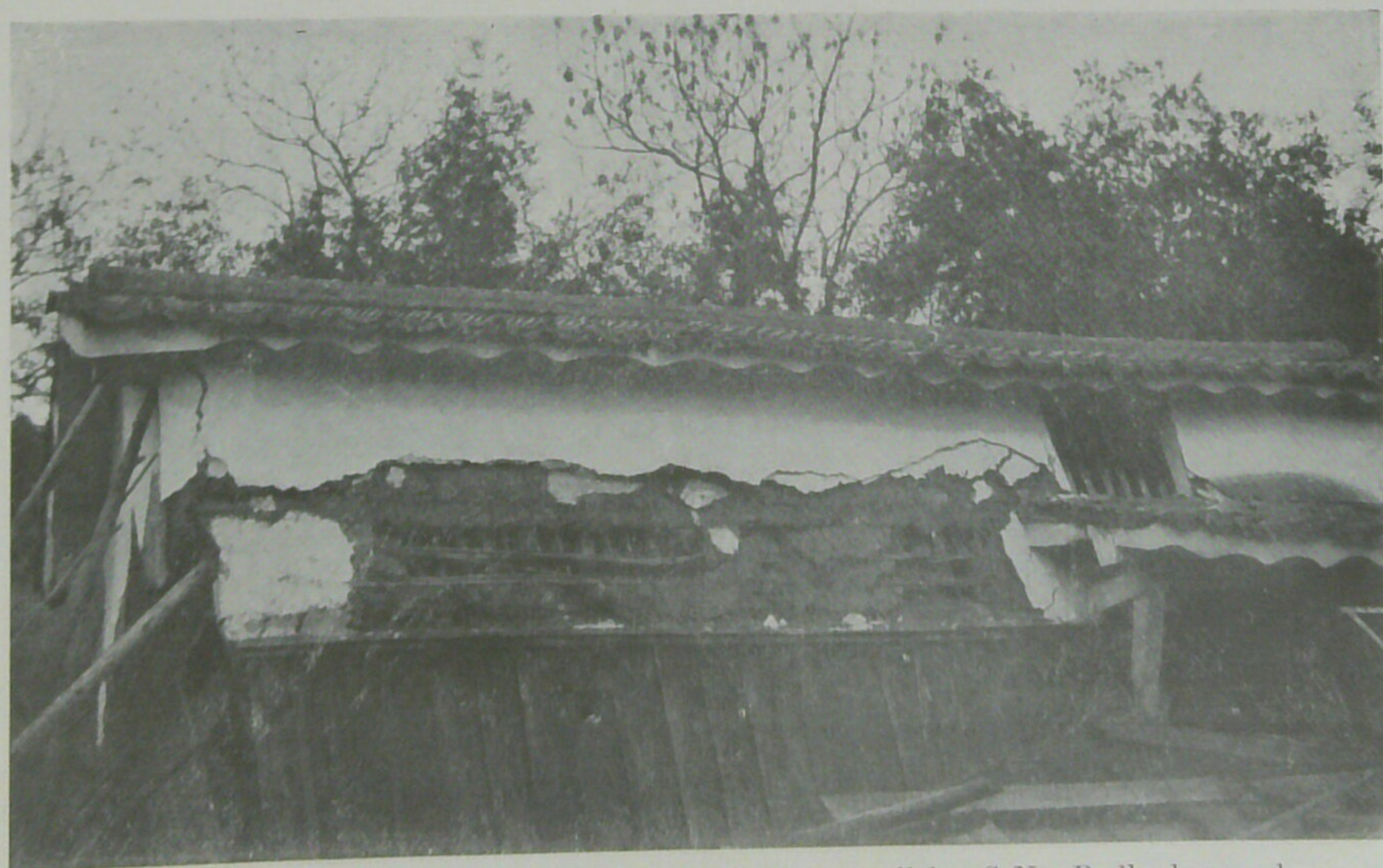
A warehouse at Kitano, Obama, with its longer side parallel to S-N. Badly damaged.
