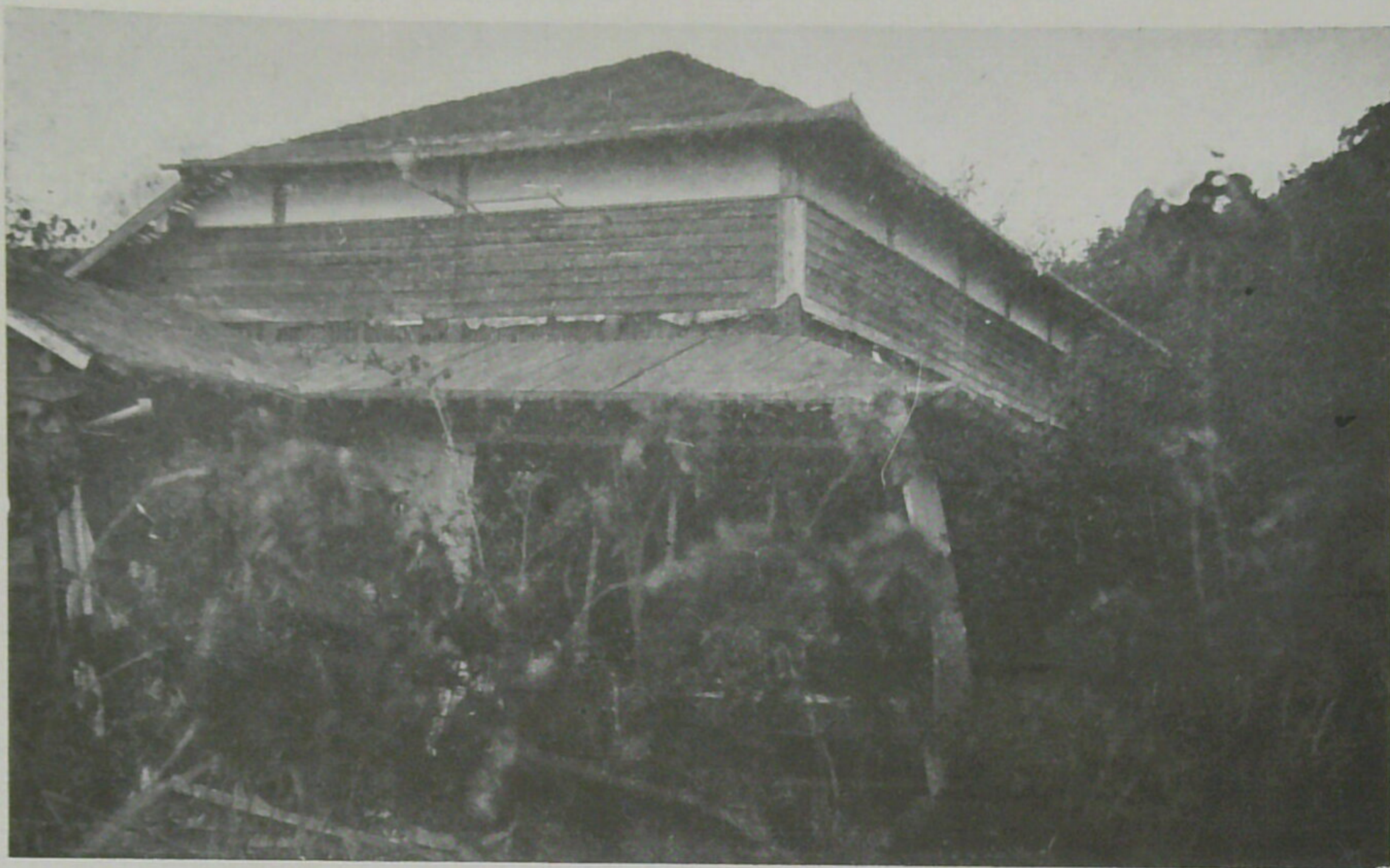
A dwelling at Kitano, Obama, with its longer side parallel to E-W. 8 pillars broken.
