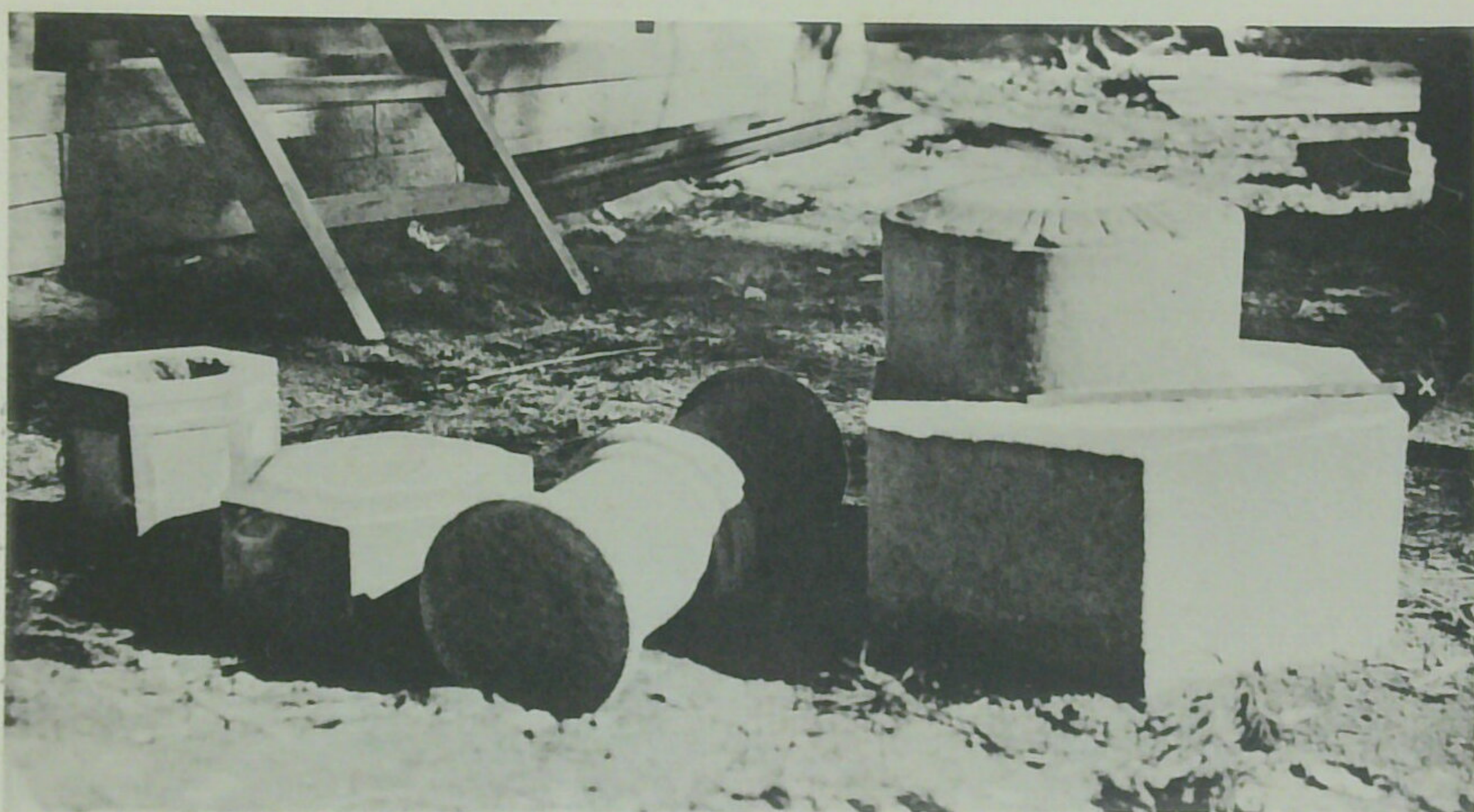
Fig. 4. A Stone-lantern overturned, at Jokoji (常光寺) Temple, Yashiro-mura. (X) ... A foot-scale indicating the amount of the displacement of the pedestal.
